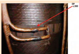
Figure 8: Showing effect of DP value<200 in a power transformer...
