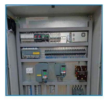
The integrated panels provide the best value for money. As we use globally renowned components like Panels from nVent HOFFMAN, Switchgear from Schneider Electric, Omron, Wires & Accessories from LAPP & Connectwell, thus adding efficiency and safety to the performance.
